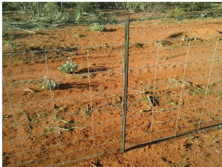
Photo 5 TGP-style fence with prefabricated mesh, constructed 1200 mm high with 50 mm ground clearance. This style of fencing is widely used throughout the wheat-sheep zone of NSW for stock control.
