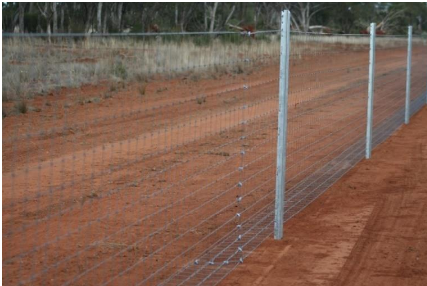
Photo 10. Exclusion fence constructed with hinged apron.
