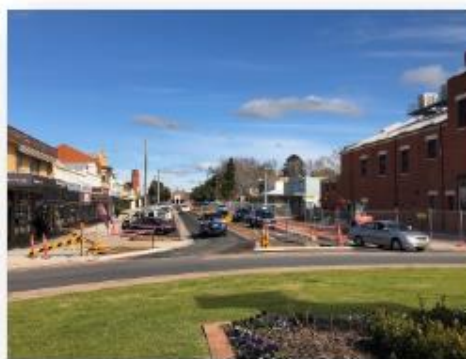
CBD Enhancement Project - Phase One Stage 1 & 2
