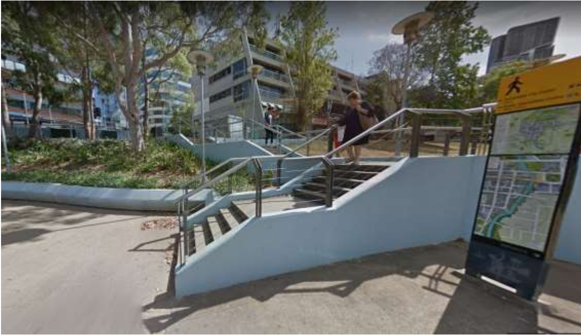
Figure 7 The Charles St Wharf is an unprepossessing introduction to the city
