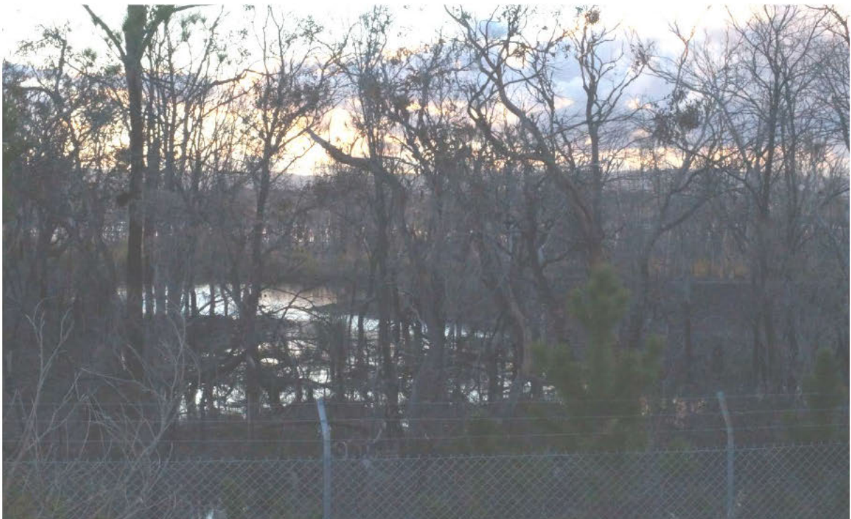
Vales Point Coal ash Dam from the Pacific Highway Doyalson NSW
