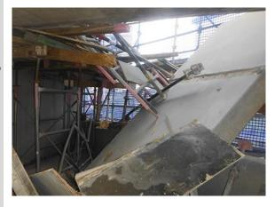
Bracing for tilt-up panels needs the input of engineers to ensure it is fit for the purpose and will perform safely without collapse and subsequent injury and damage. Without a compulsory registration scheme for engineers that applies beyond Class 2 structures, vital areas of engineering will remain at risk.
