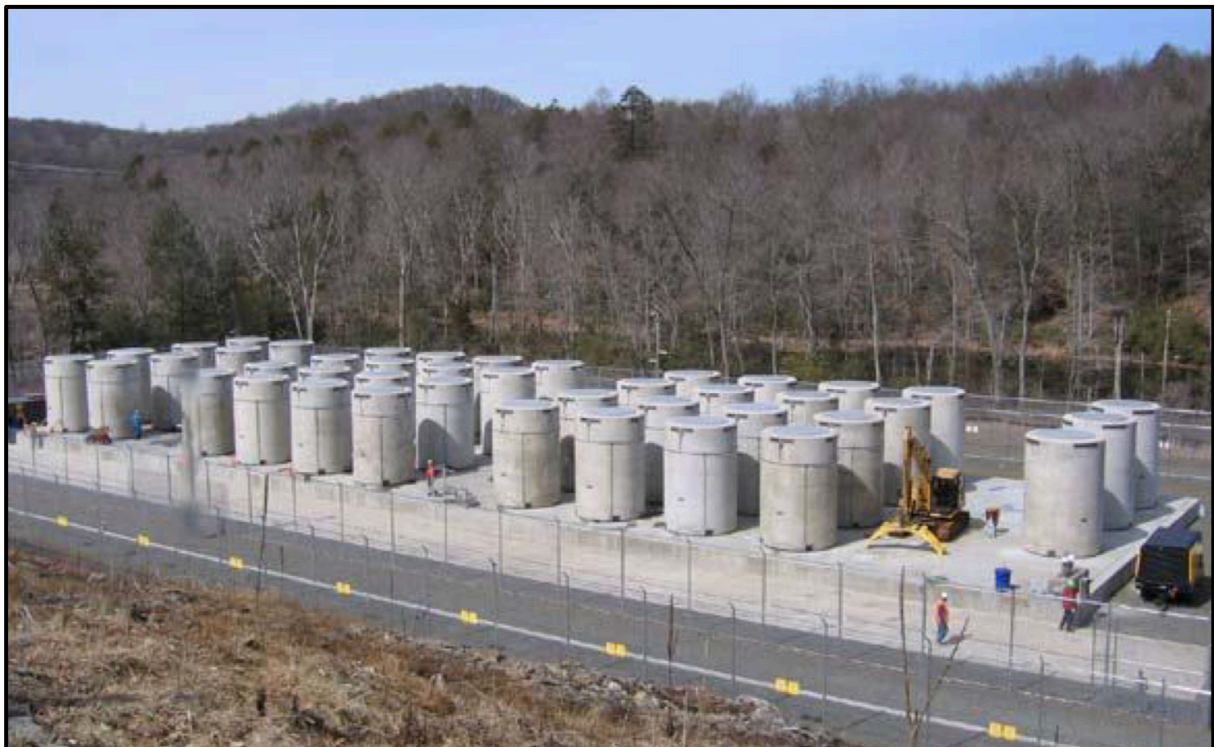
Figure 3 - Dry cask storage at decommissioned Connecticut Yankee Nuclear Power Plant
