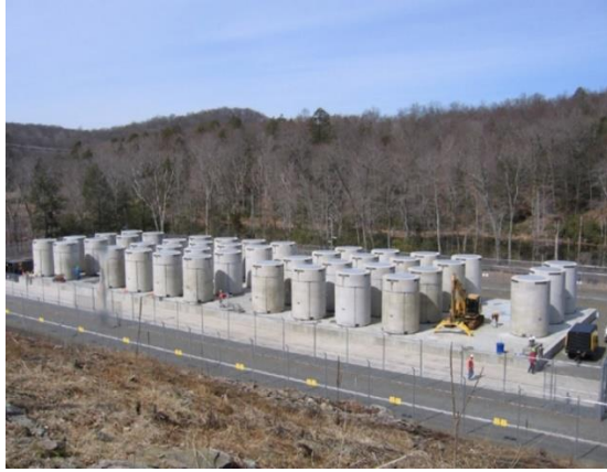
Figure 4. SNF in dry casks is shown here at the Connecticut Yankee nuclear power plant site. This storage area is all that is left of the now decommissioned nuclear plant, which generated 580 MW of electricity for 21 effective full-power years. We estimate that if SA were to use nuclear power at 1000 MW (thus providing about 75% of SA's total electricity demand) for 40 effective full-power years, the total number of dry casks accumulated would be about 140 (source: http://www.connyankee.com/html/fuel_storage.html )
