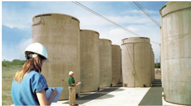
Figure 5. Dry casks containing spent nuclear fuel are inspected at an unspecified US nuclear power plant. The cask design includes radiation shielding, so that approaching and handling these casks exposes the workers to a negligibly low radiation dose. (source: Nuclear Energy Institute)
