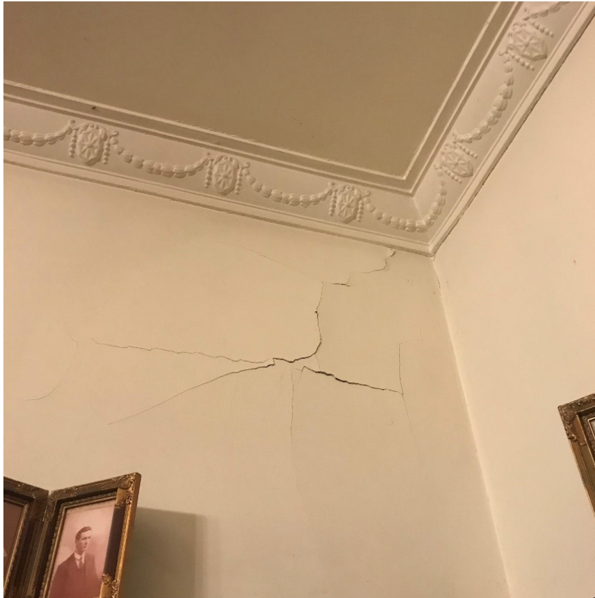
Figure 2 - another sheet of plaster soon to collapse.
