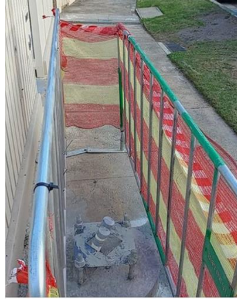
Photo 3 VMS foundation in Dalhousie St
