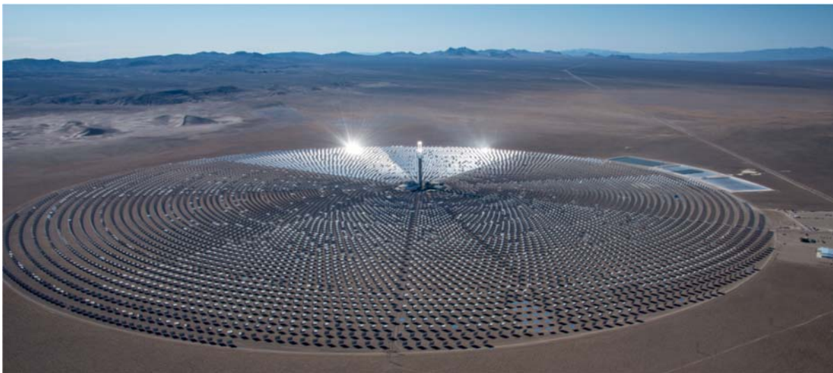
Crescent Dunes Solar Energy Project, Nevada, USA. 110MW with 10 hours of full load storage (1,100MWh)
