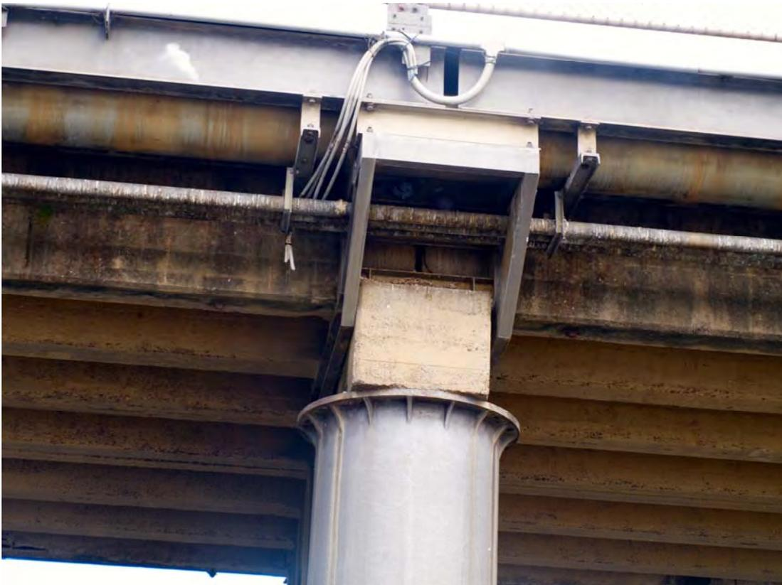
PHOTO C: END OF FABRICATED STEEL CANTILEVER – NOTE SUPPORT RSJ'S FOR FOOTWAY
