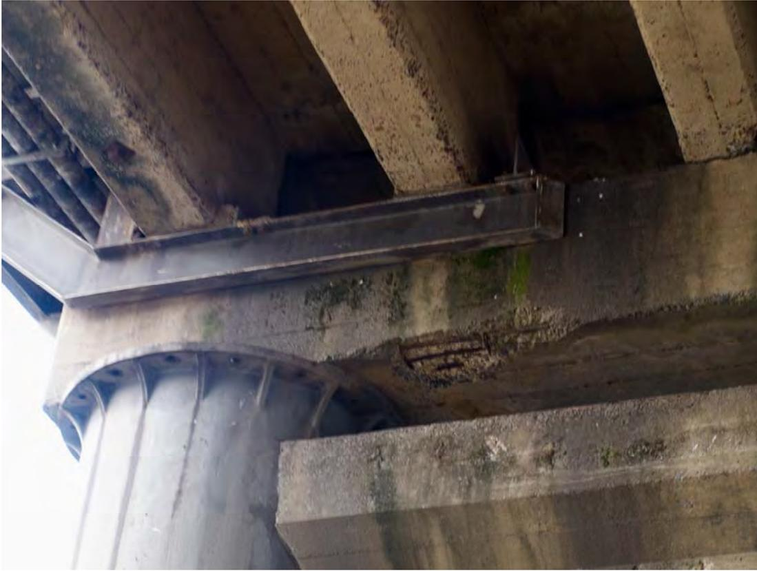
PHOTO B: FABRICATED STEEL MEMBER BOLTED TO PIER HEADSTOCK
