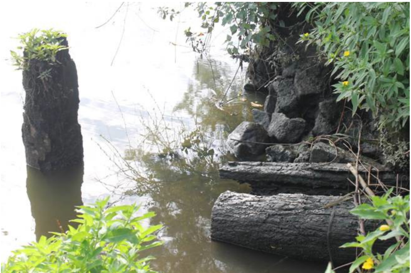
Photo 4a. The 2 walers near the solitary pile.
