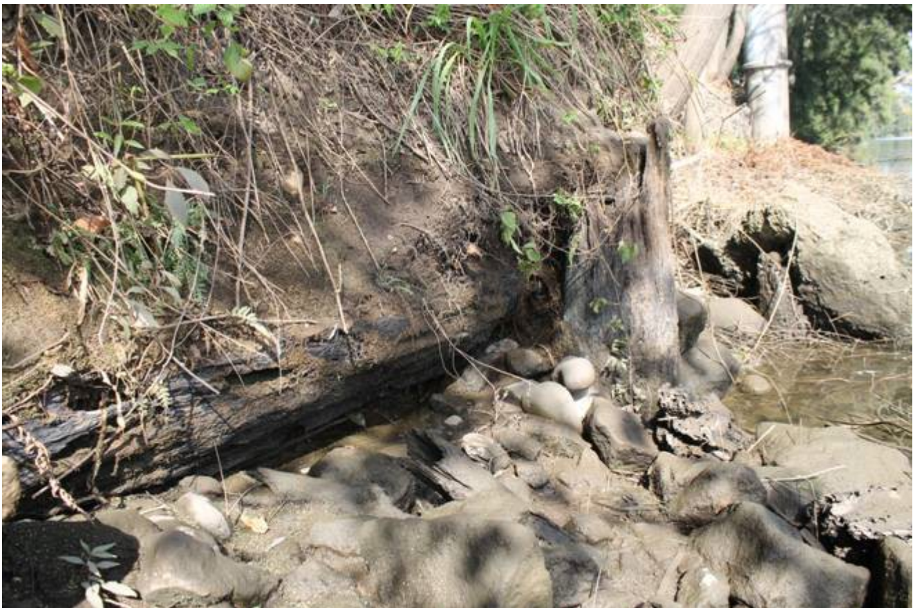
Photo 10a. This appears to be the most western pile attached to any beams, the pile next to the concrete (photo 9c) is smaller and lower, and the fill angles back toward the bank per photo 10. The southern bridge pylon is visible in the background.
