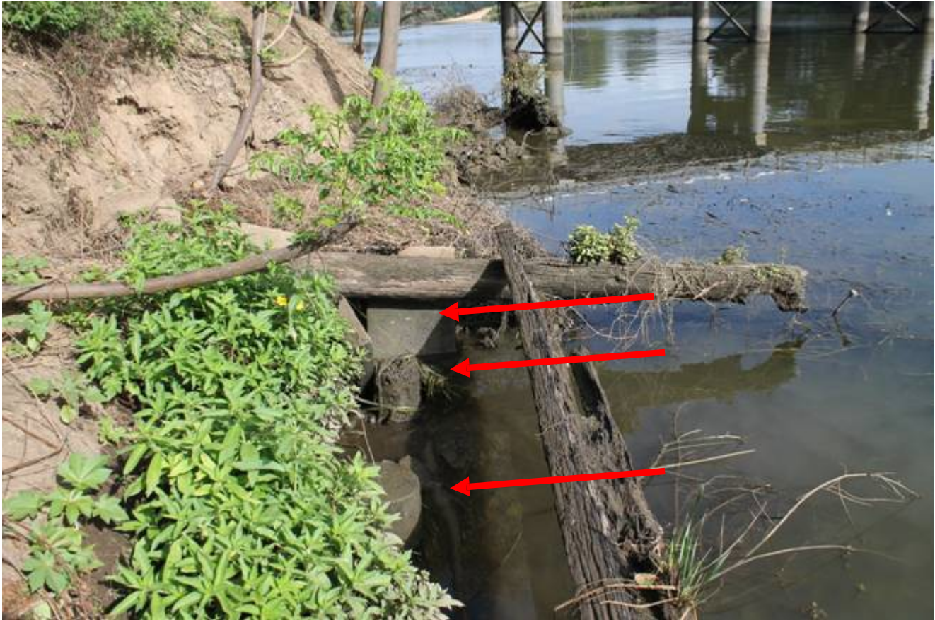
Photo 6a showing 2 piles spaced 3 feet apart as per contract, and sandstone slab between walers. There are 2 other sandstone slabs buried under the pile of weeds at the west adjacent to these remains (top end of picture)
