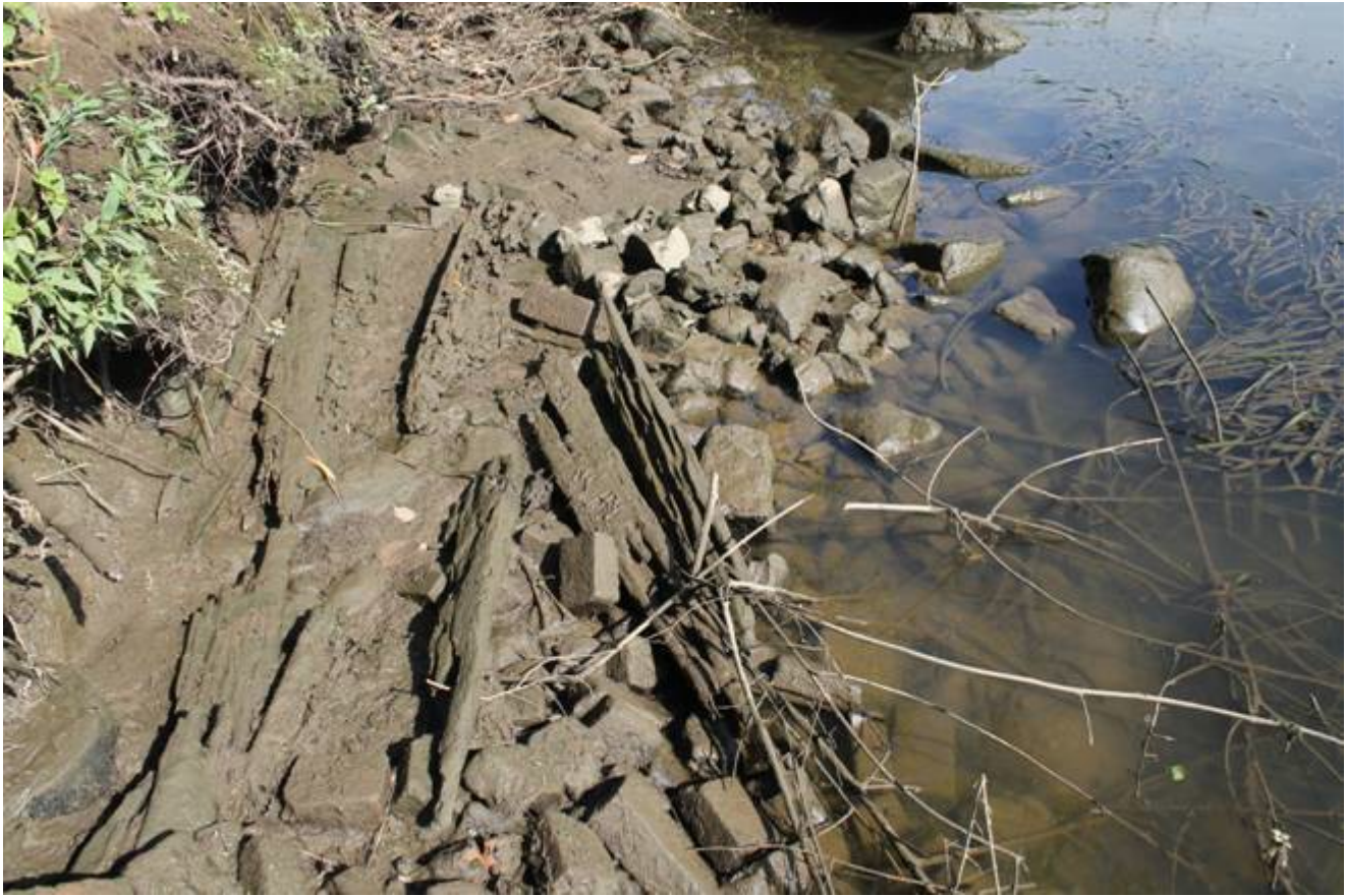
Photo 7c. Wharf deck timbers on river bed. Remains of a beam are contained in the bank.
