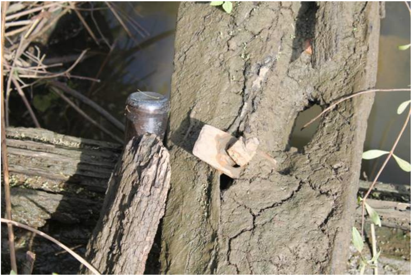
Photo 6c closer image of iron fastener through Waler and beam
