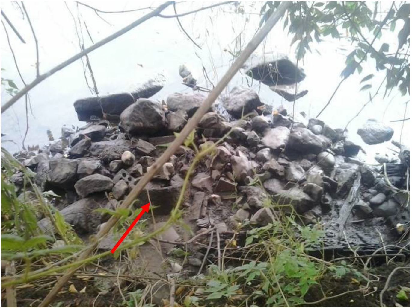
Photo 7h 1/3/2018. Note concrete pipe fragment appears to be consistent with that located at the "end" of the barrel drain, and wharf timber bottom right. Modern bricks and other fill in general area.
