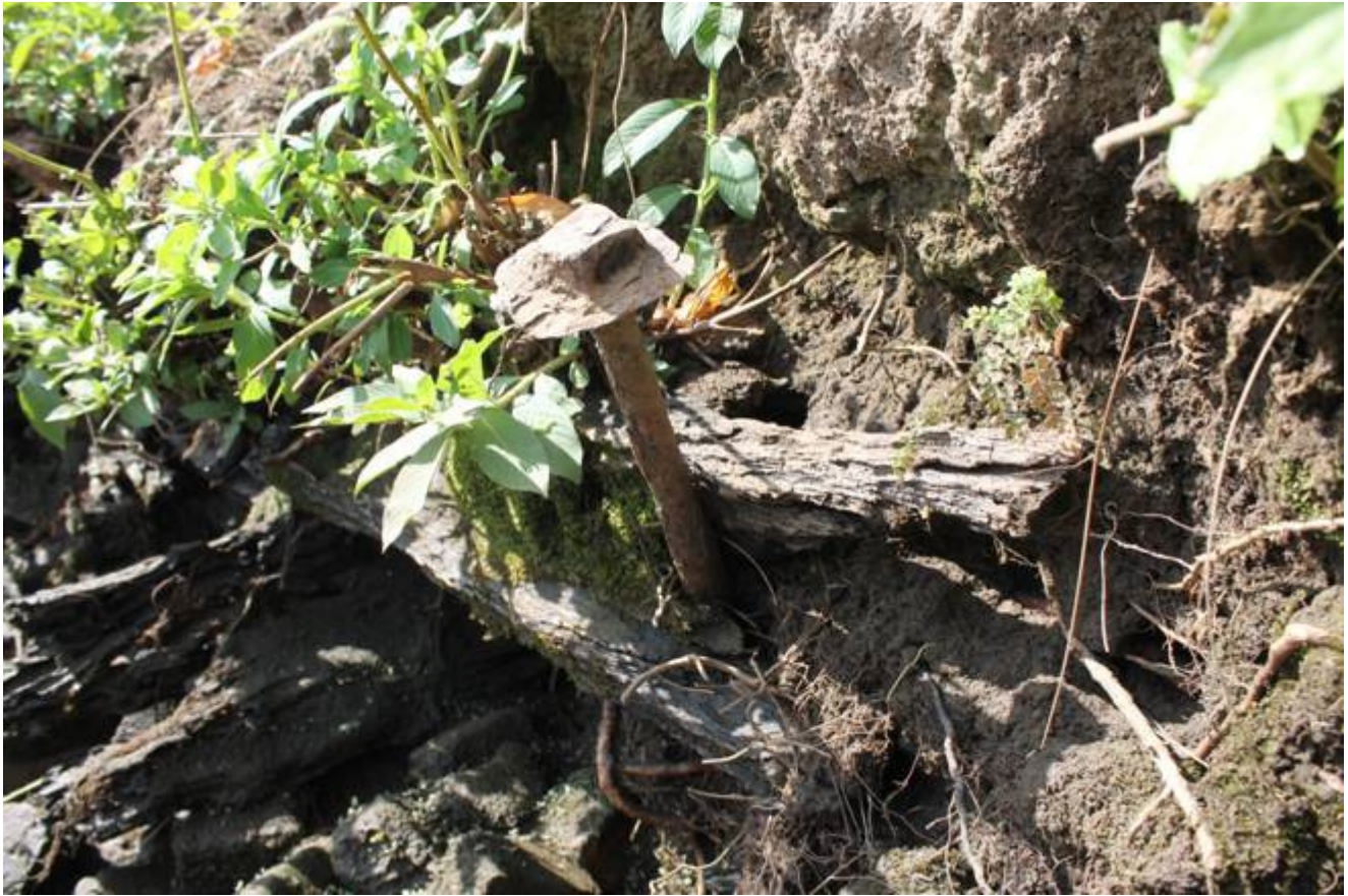
Photo 7e. Iron fastener in remains of beam in bank.
