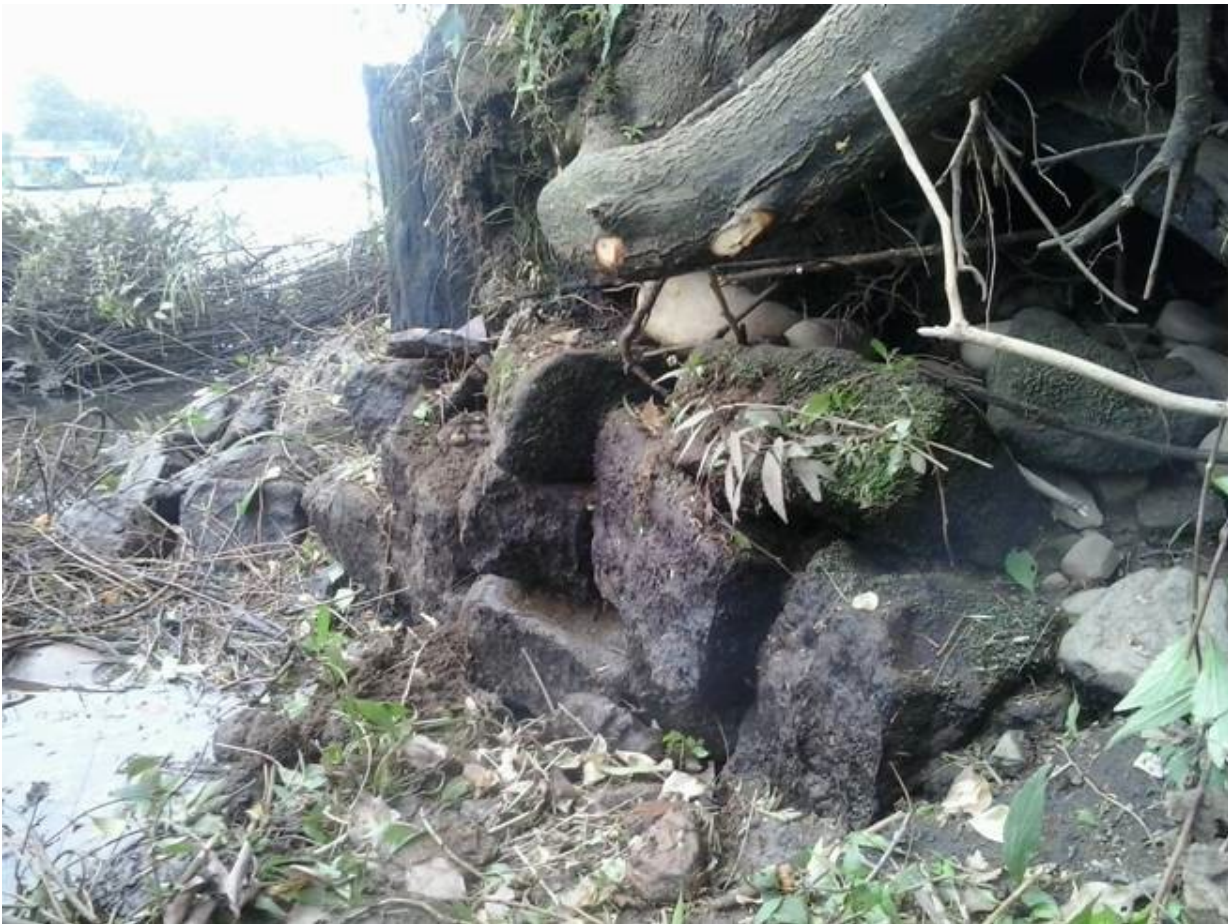
Photo 10 3/4/2018. Scour protection at western end of wharf, pile at left of looped tree root.
