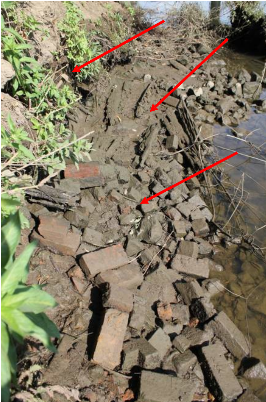
Photo 7. Bricks consistent with barrel drain, wharf deck timbers and an iron fastener, to the west of the above water wharf remains. Most of this is visible only at low tide. Brick position consistent with estimated drain outlet.
