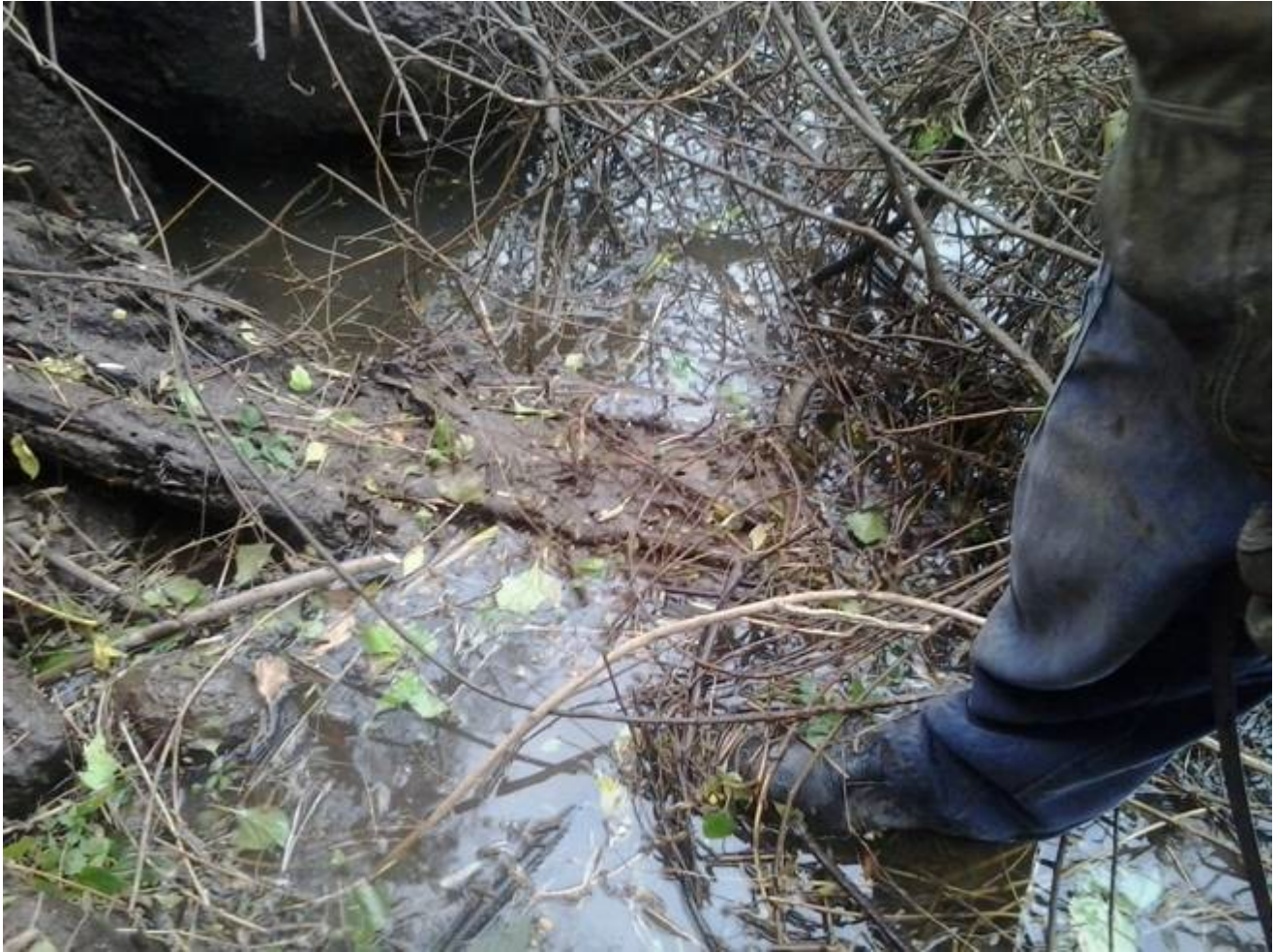
Photo 9b 3/4/2018. Rotted beam in water disintegrated due to weight of iron fastener in one end.
