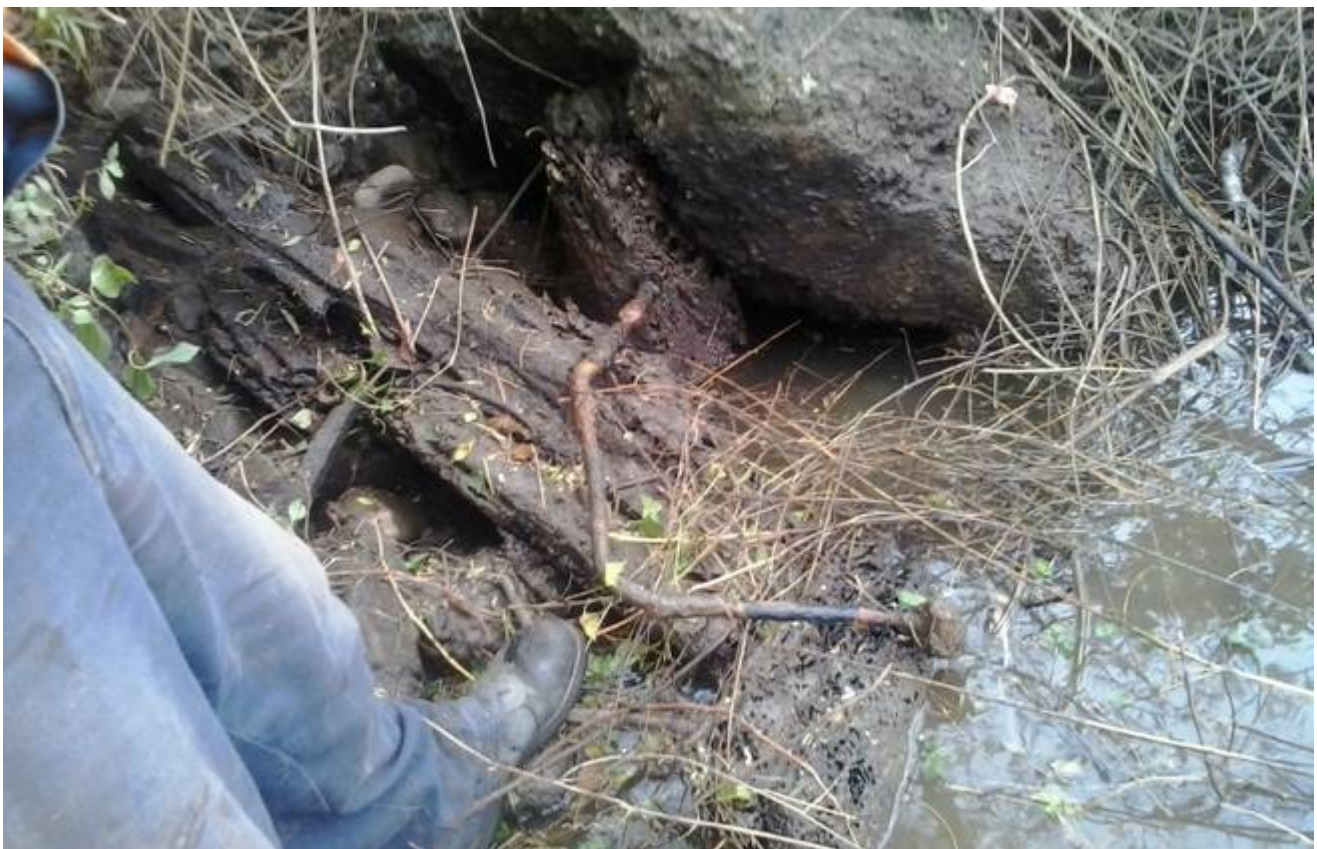
Photo 9d 3/4/2018. Iron fastener, now held by Hawkesbury Museum. Disintegrated beam under iron.
