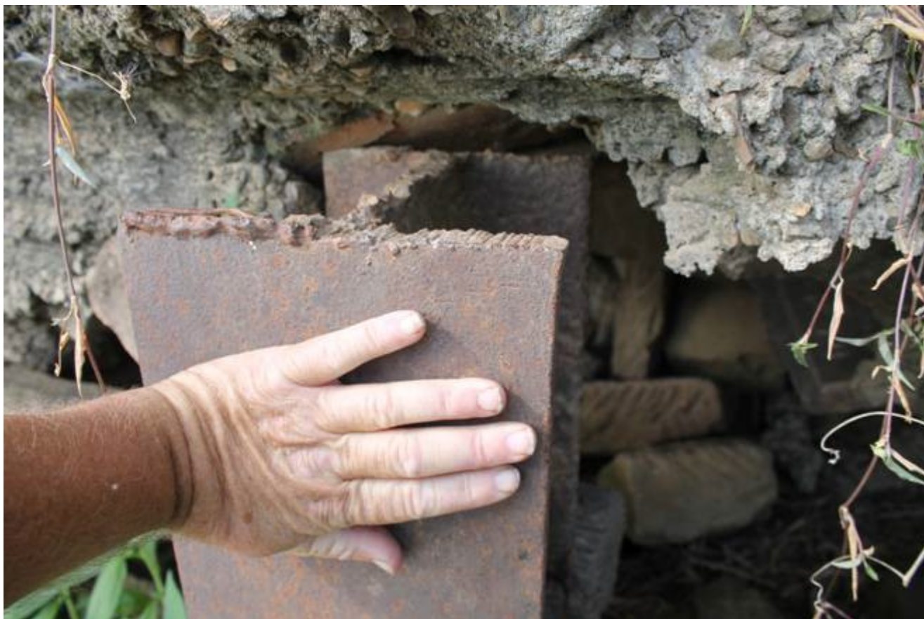
Photo 2c. Beams holding retaining wall are 20cm wide, clearly not square.
