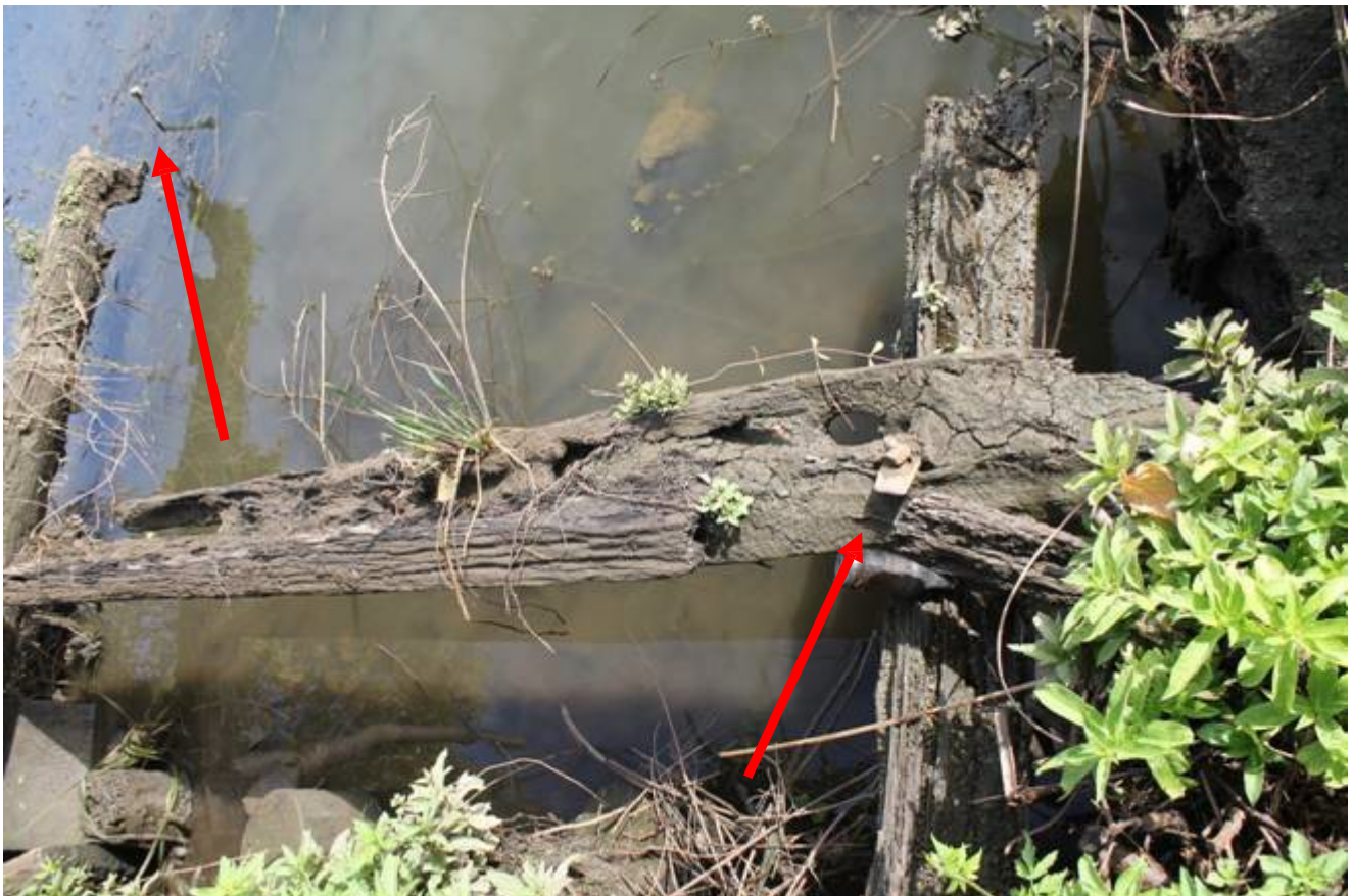
Photo 6. Above water remains showing 2 iron fasteners (and a beer bottle).
