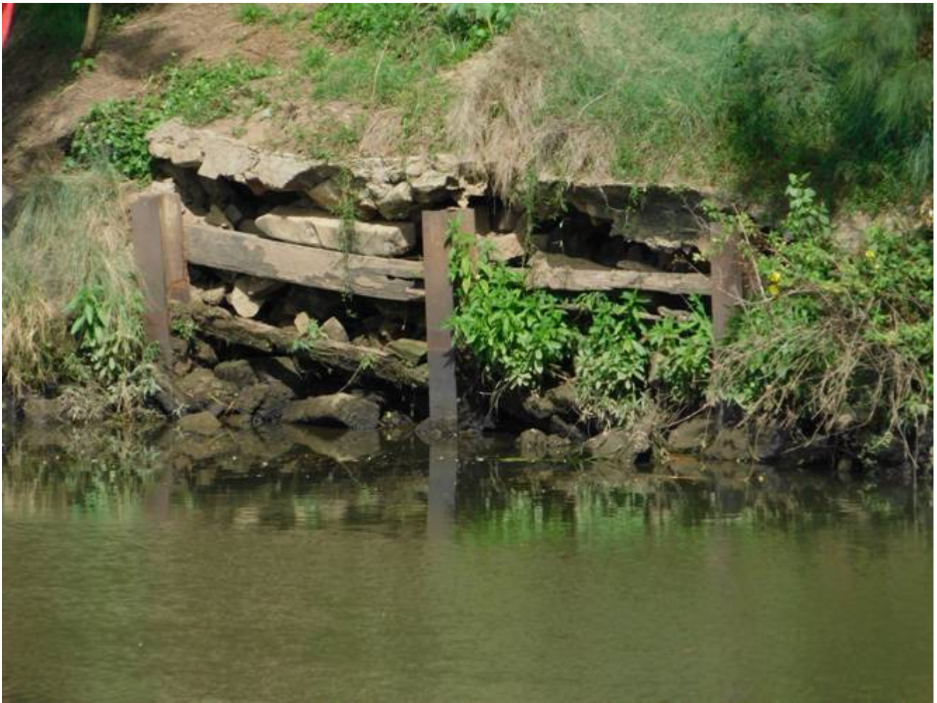
Photo 2a. The retaining wall viewed from the northern bank, showing the concrete capping
