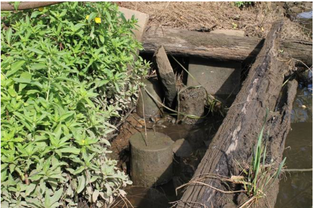
Photo 6b showing closer shot of piles (third now visible). These piles were not mentioned by Cosmos.
