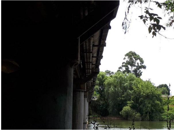
Fixtures/fittings attached under the current bridge showing potential for flood water debris to damage or get caught up in.
