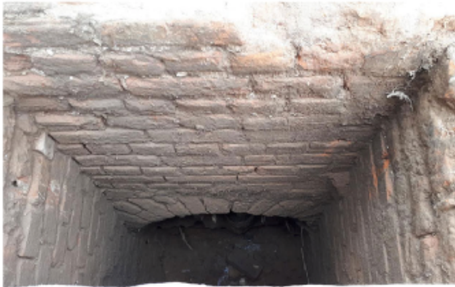
Brick barrel drain pumped out
