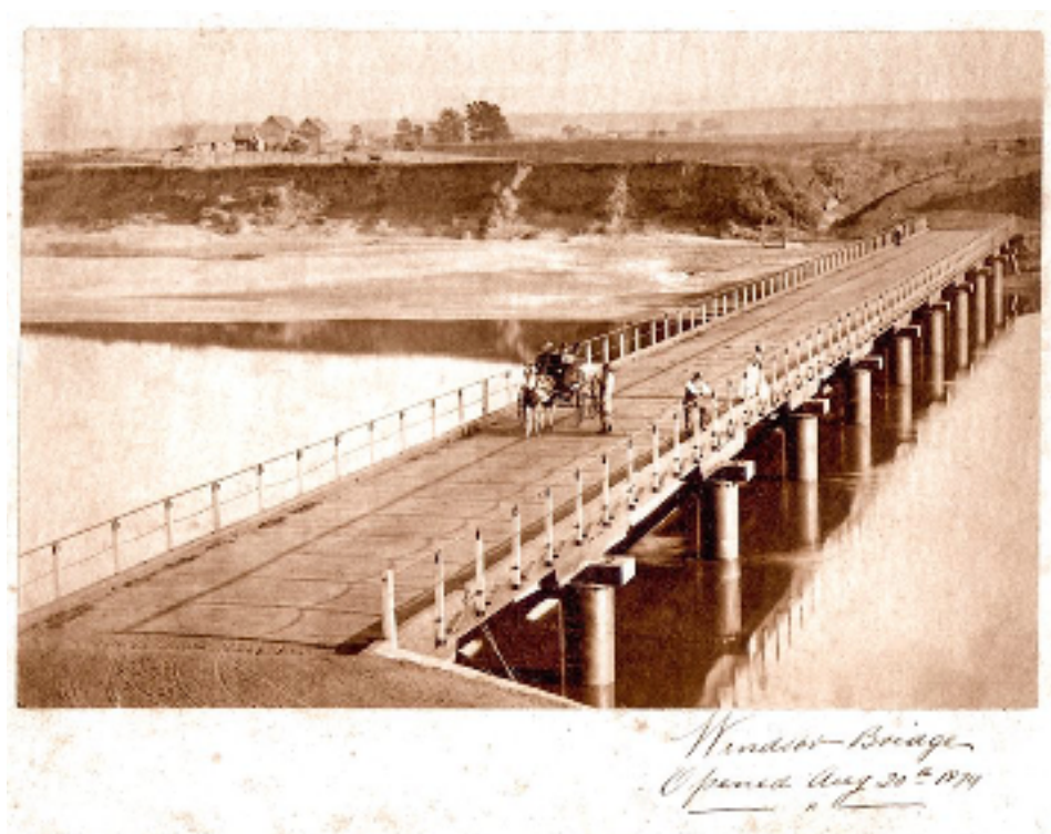
Figure 1. The Windsor Bridge with the original deck
