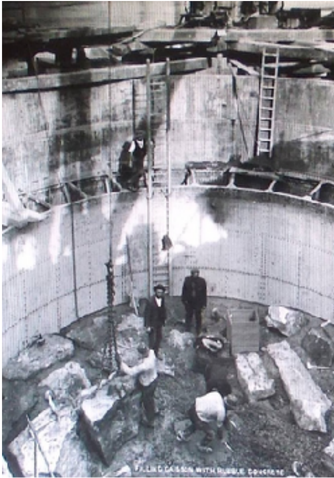
Figure 2. Caissons constructed for the Pyrmont Bridge, NSW. Figure 3. Caisson; devised 1846, Jules Triger
