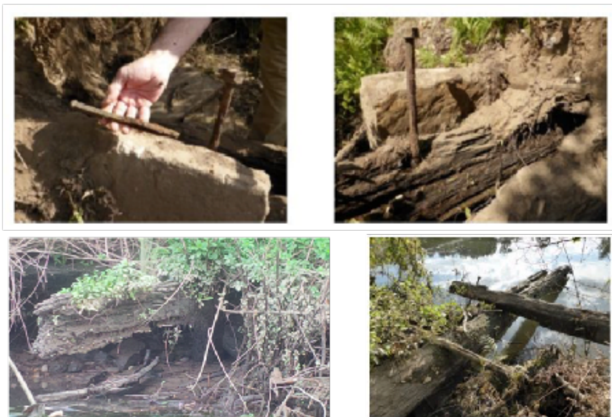
Figure 31. Wharf remains currently visible.
