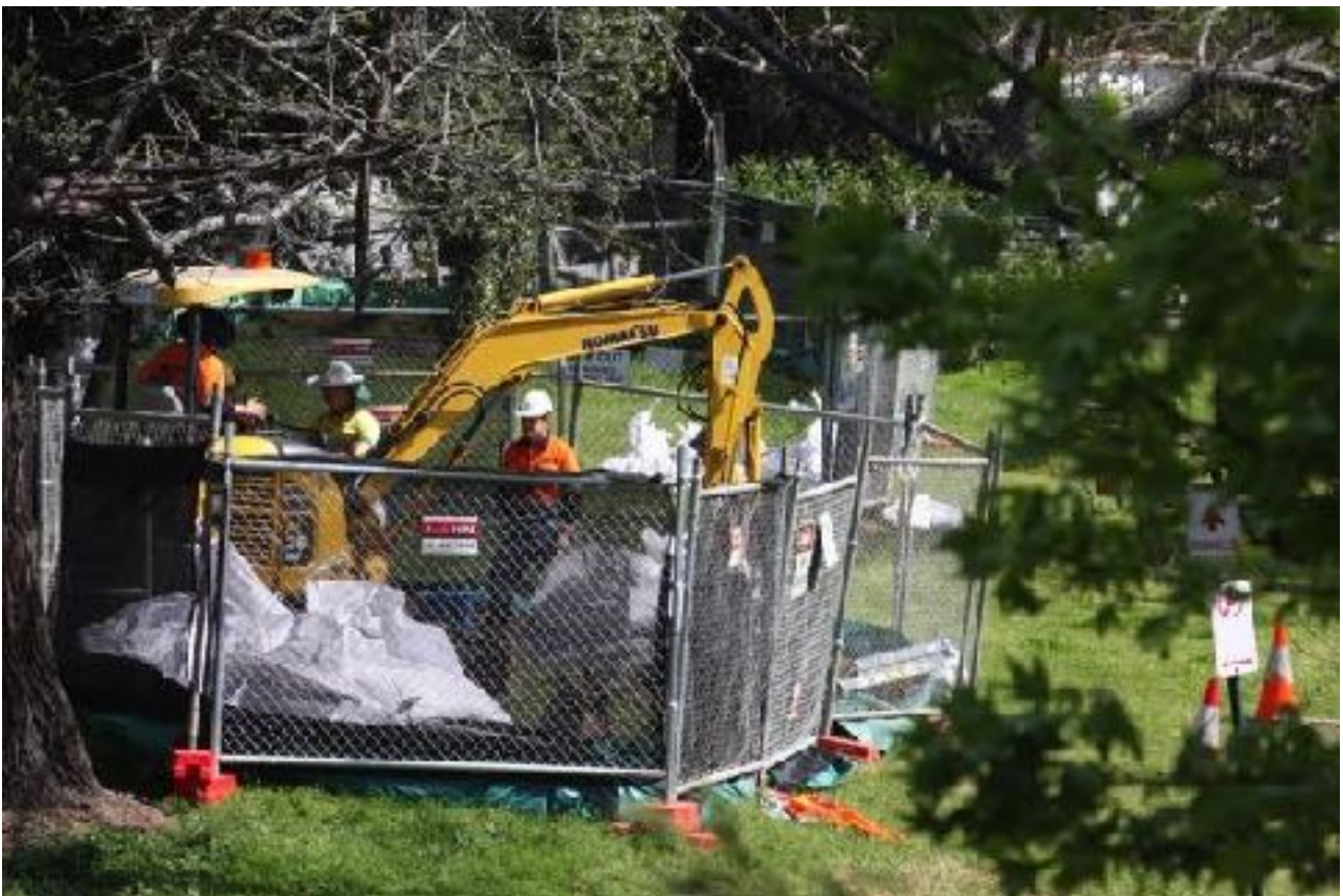
16/9/16 - A series of pictures showing the digger filling the white bags held by two workers
