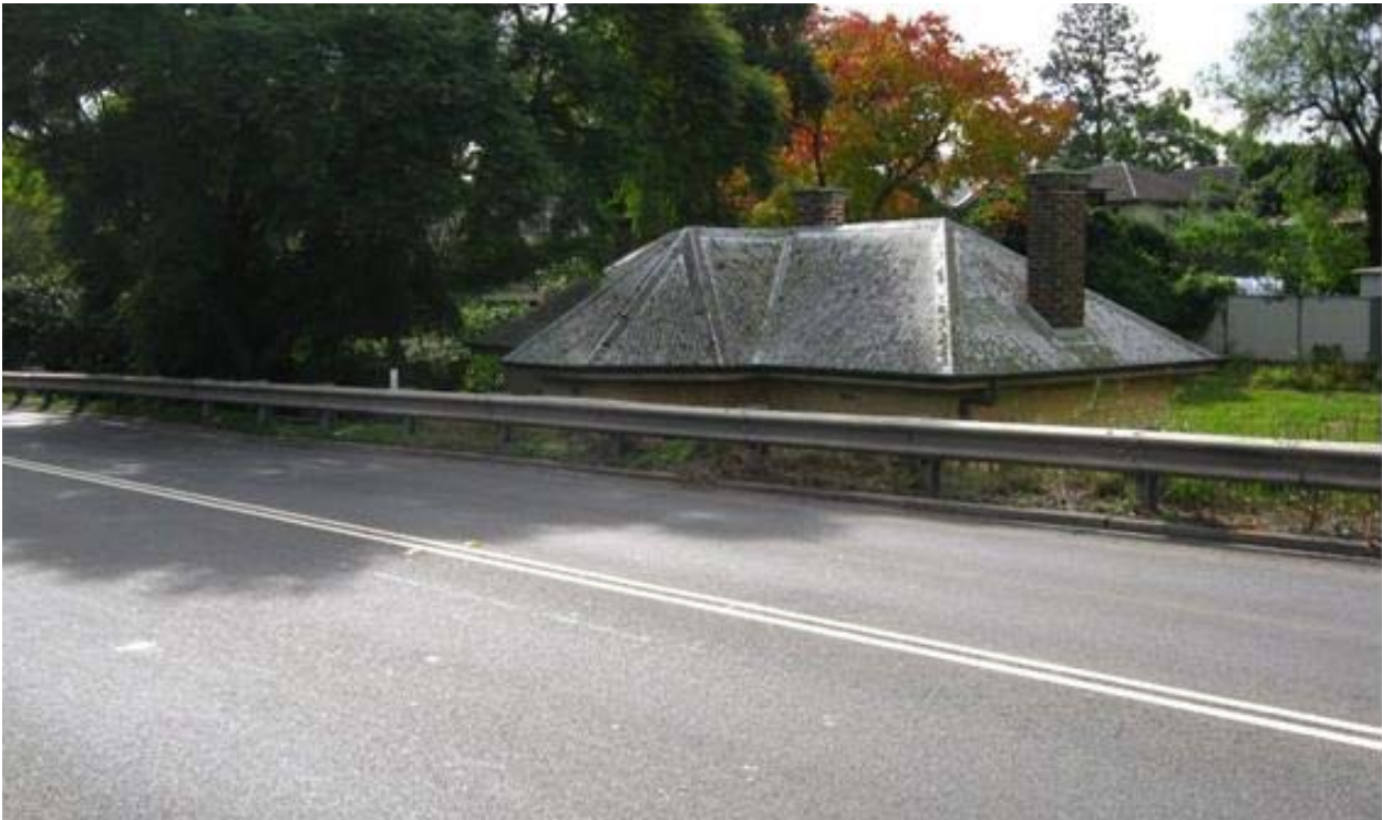
The Windsor Toll House, at the Fitzroy Bridge crossing over South Creek at the entrance to Windsor, one of only 2 remaining intact Toll Houses in NSW, after the raising of the Fitzroy Bridge
