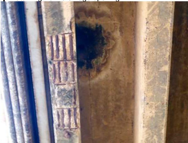
↑ Exposed reinforcement near drain
