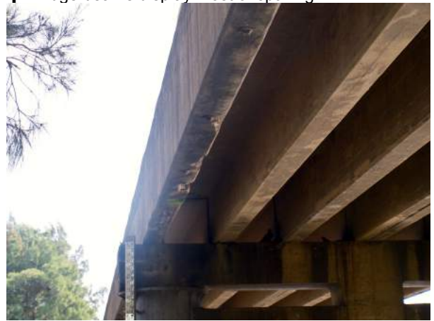
↑ Note good condition of interior beams
