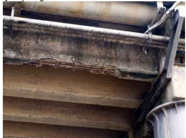
↑ Edge beams display most of spalling
