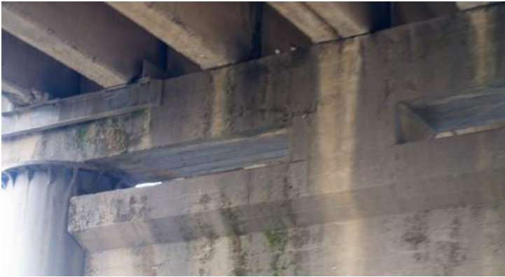
↑ Note joint between central beams
