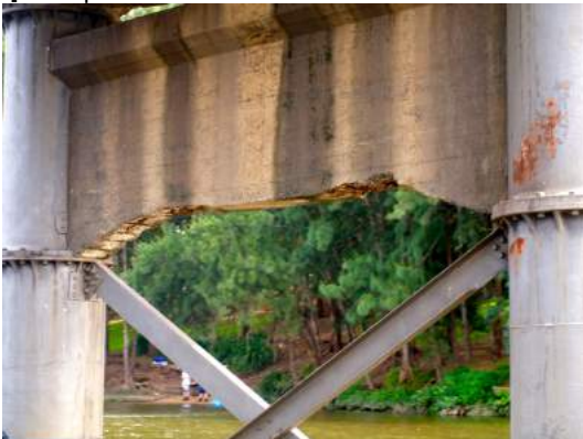
↑ Diaphragm at pier bracing
