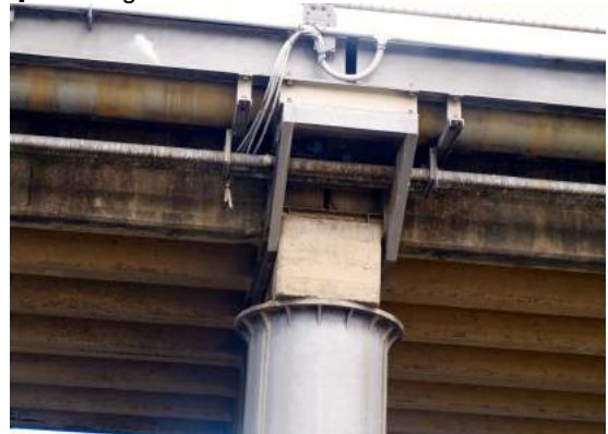
↑ Note interior beams in good condition
