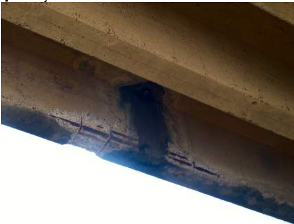
↑ Staining from drainage opening
