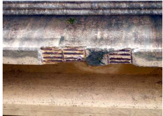
↑ Spalling of concrete due to corrosion of reinforcement
