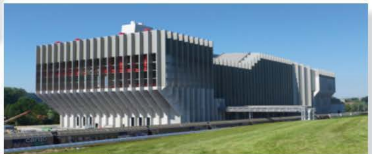
Lucerne Switzerland (2015) Net Electricity Production – 18MWe Process steam to paper mill – 22MWth R1 = 0.75 Savings in CO_2 – 450kg/t
