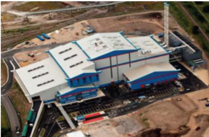
Cleveland UK (2013) Thermal power per line: 2 x 46 MW Electric power output 26 MW (gross) R1 = 0.70
