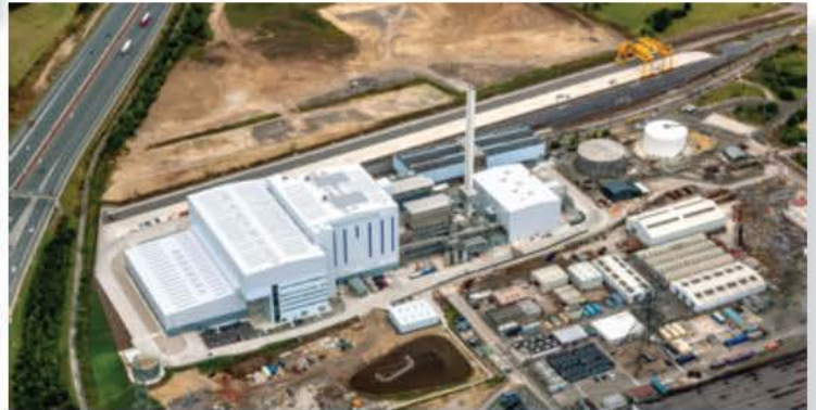
Ferrybridge UK (2015) Net Electricity Production – 67.8MWe Net Electrical Efficiency > 31% R1 = 0.85 Savings in CO_2 – 670 kg/t waste
