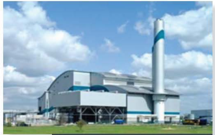
Riverside UK (2013) Thermal power per line: 3 x 81 MW Electric power output 73 MW (gross) R1 = 0.81
