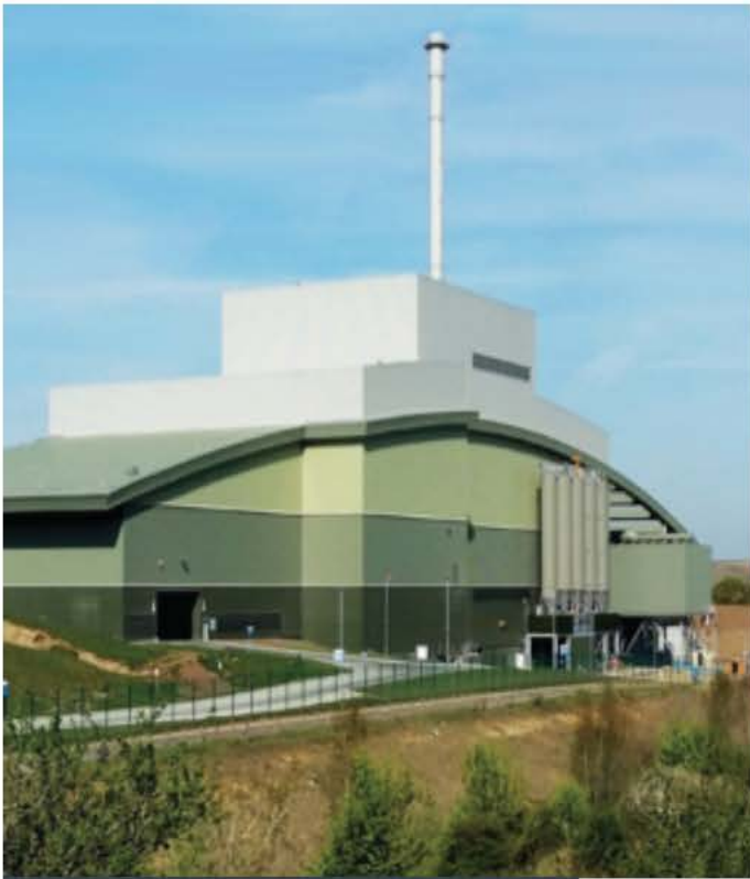
Buckinghamshire UK (2016) Thermal power per line: 1 x 101.8MW Electric power output: 29.4 MW District heating output: 6.6 MWth www.greatmoor.co.uk/emissions-reports/
