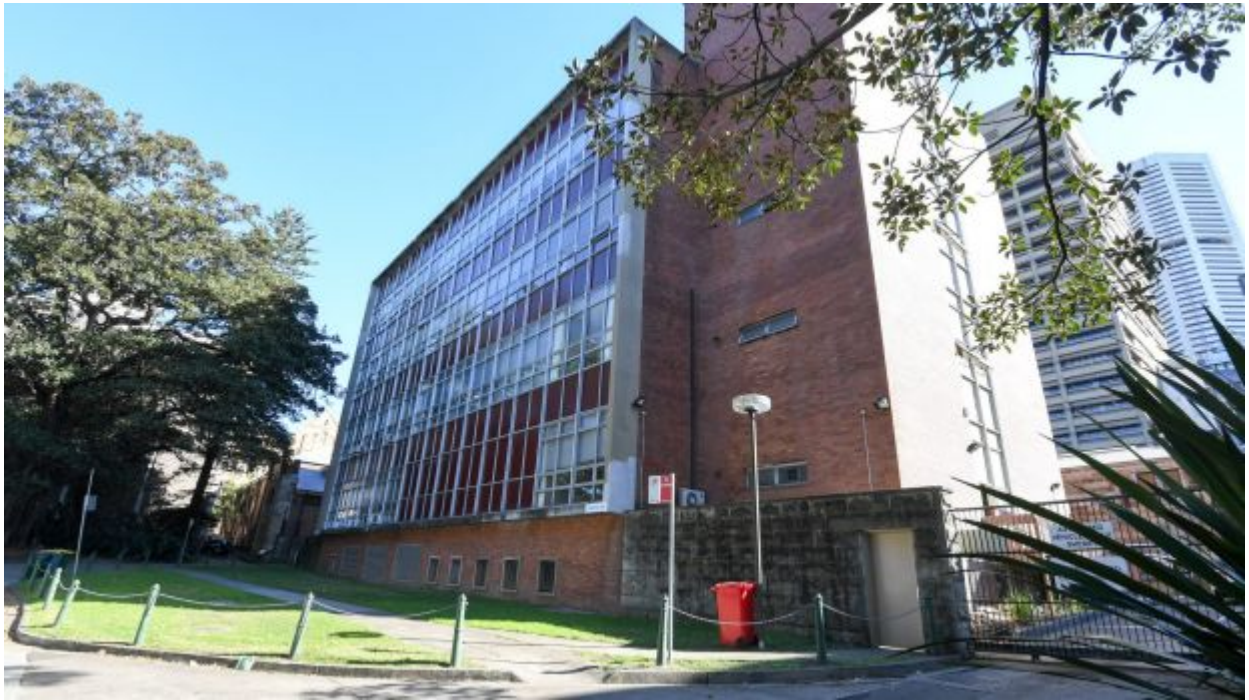
The court building facing Hospital Road and the Domain is earmarked for demolition. Photo: Peter Rae
