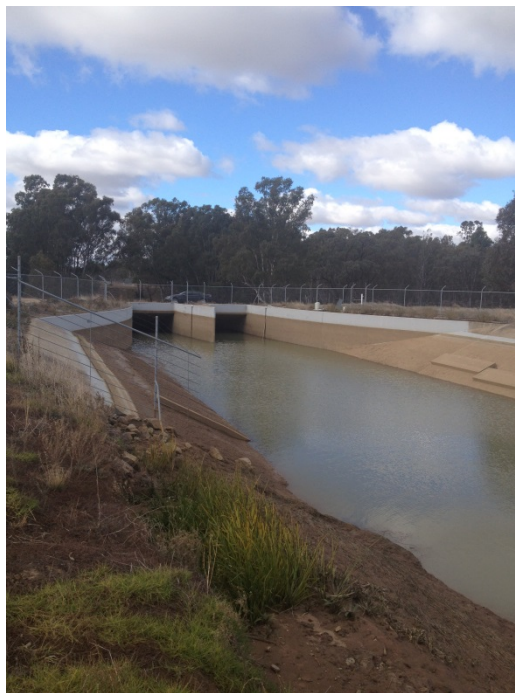
Picture of Mulwala Canal entering a Lawson Siphon under Aljo's Creek, Deniliquin NSW
