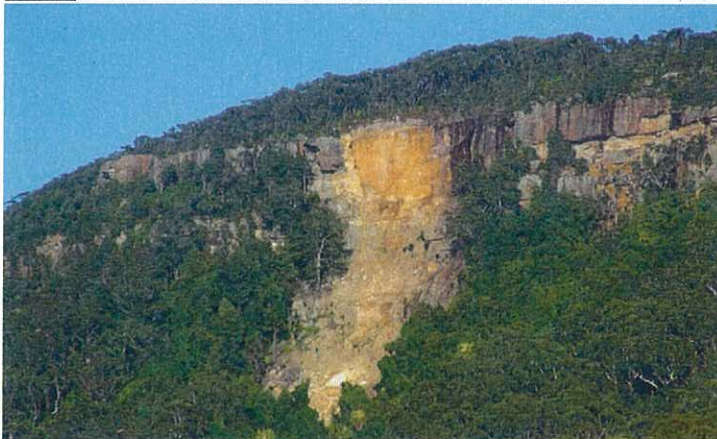
PHOTO: RECENT SLIP ALONG THE FACE OF THE ESCARPMENT AT WOMBARA
