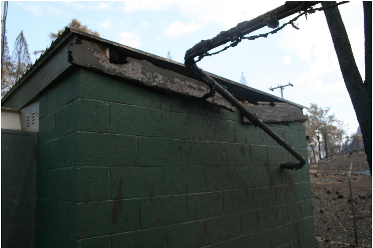
Damage to water pumping station
