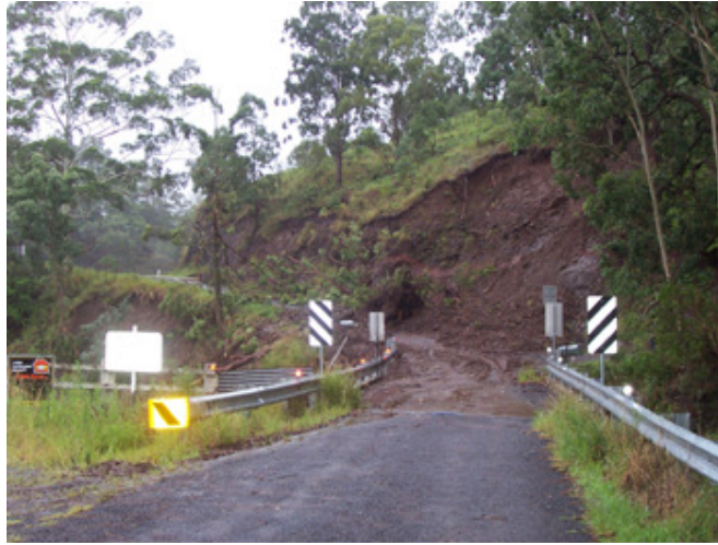
Figure 3: Landslip on the Lions Road
