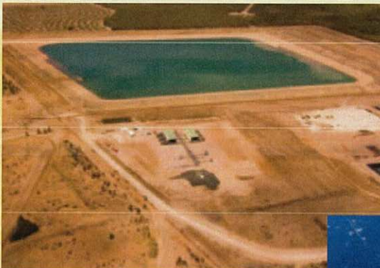
Waste water evaporation pond and compressors
