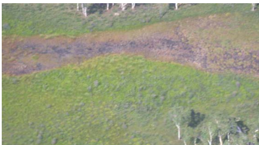
Figure 3. Scalding in an Upland Swamp on the Woronora Plateau, upper end of Lizard Creek, as a result of alkaline mine water discharge. [162]
