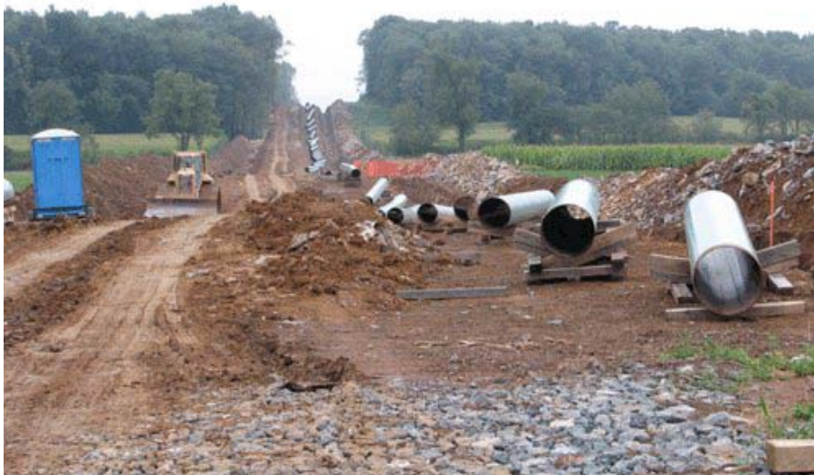
Figure 11. Land clearing and the laying of gas pipeline.
