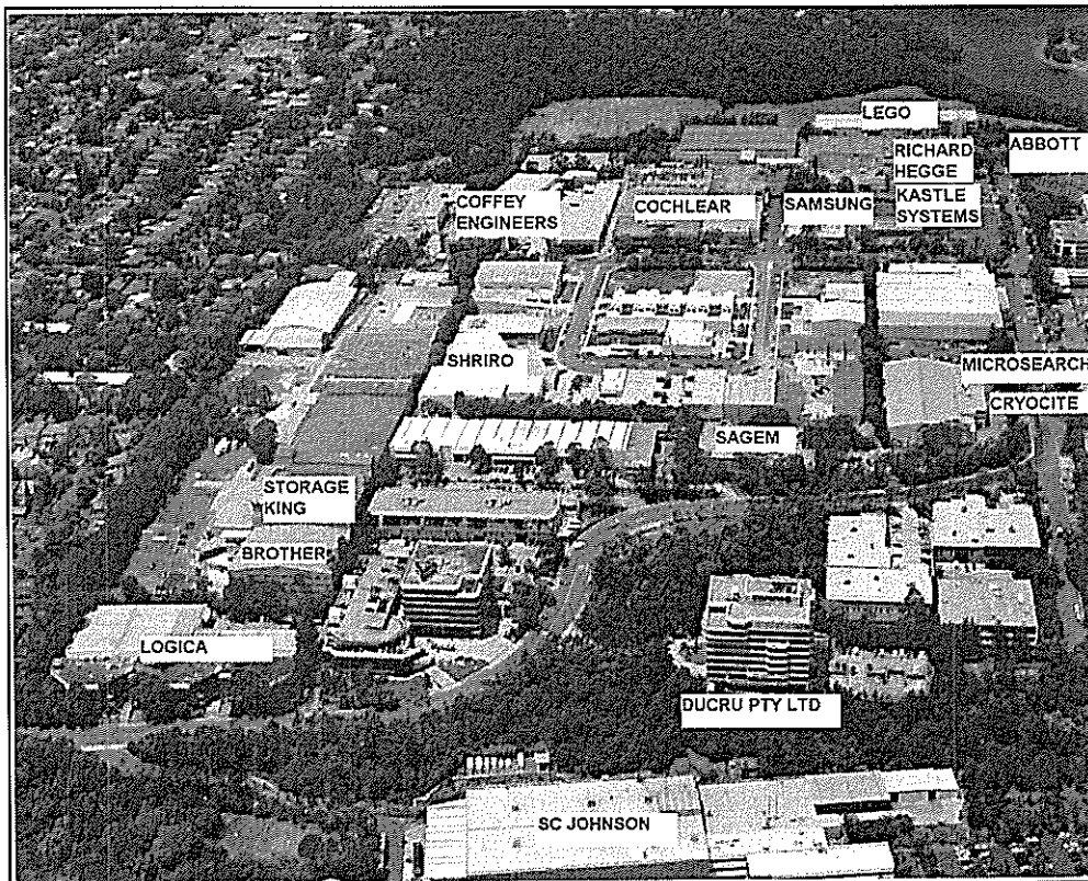
FIGURE 2: ESTABLISHED BUSINESS PARK
