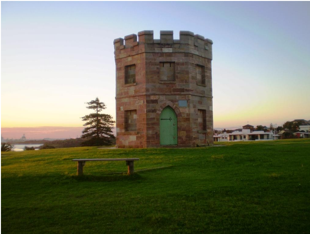
*Macquarie Watchtower – the first ‘customs house’ in Australia built during Governor Macquarie era (photo taken prior to ‘renovation’).
