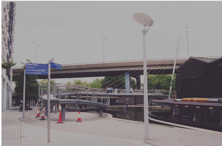
Pedestrian and bicycle bridge over the canal next to Paddington railway station, London
