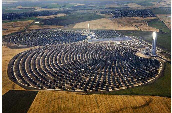
The PS10 11 Megawatt Solar Thermal Power Plant located 25 km west of Seville in Southern Spain. The solar radiation, mirror design plant is capable of producing 23 GWh of electricity which is enough to supply power to a population of 10,000.
