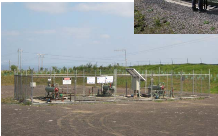
WELL PAD WITH THREE HORIZONTAL WELLS Photo courtesy of AGL
