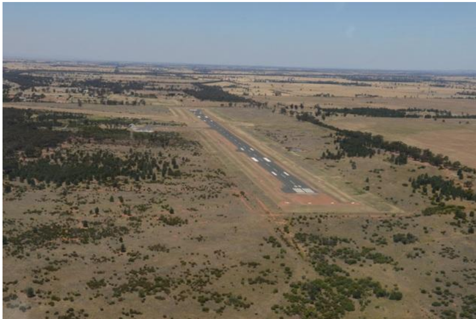
West Wyalong Airport
