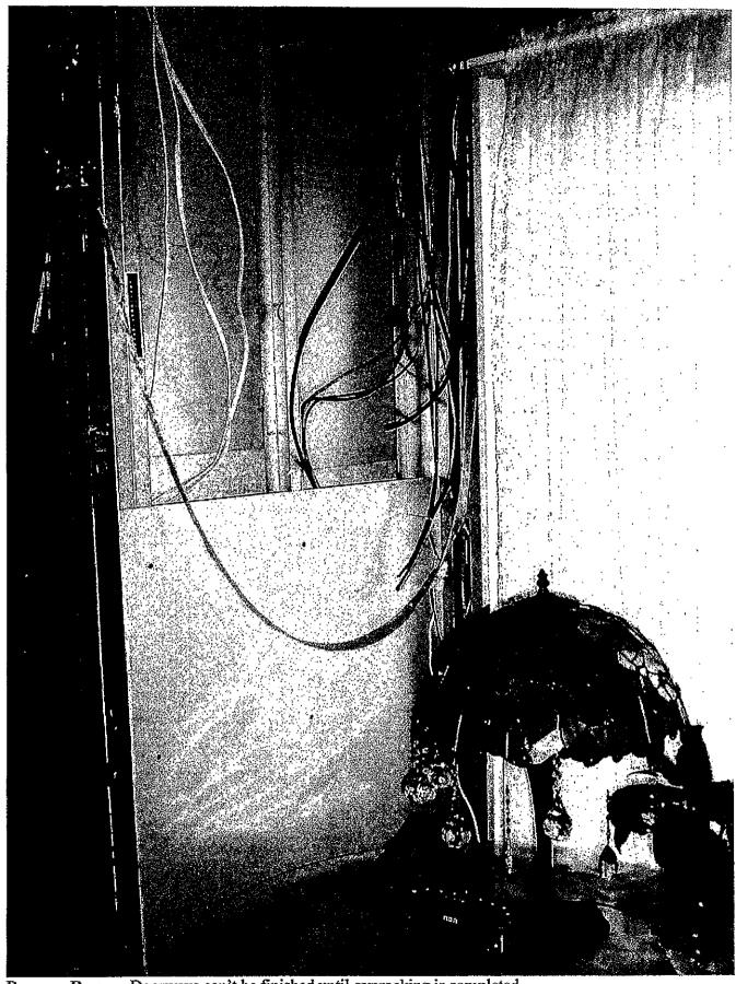
Rumpus Room Doorways can't be finished until gyprocking is completed Data and TV cabling is shown –similar cable sets are in every corner of every room.
