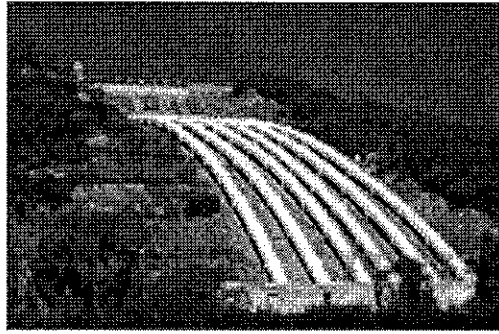
Tumut 3 Power Station (Source: www.snowyhydro.com.au )
