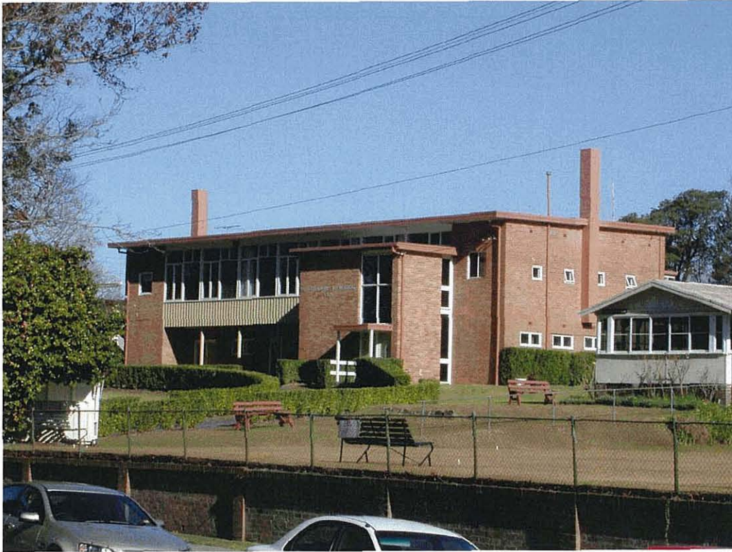
Above Photo: The completed site showing the two false chimneys
