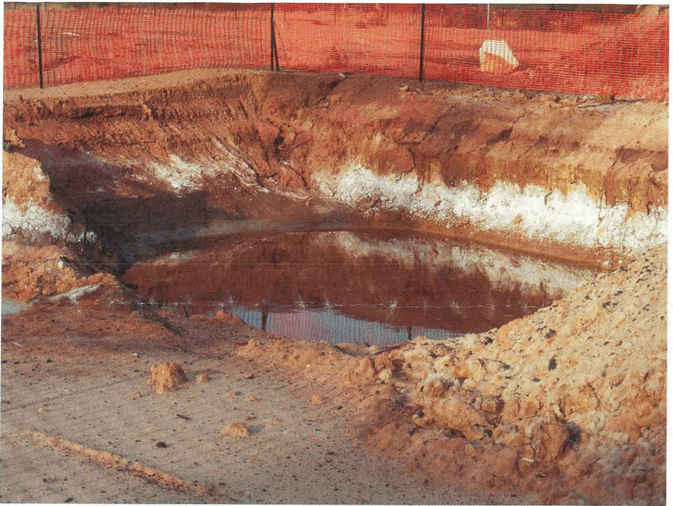
Above: Produced water from CSG operation and saline crust formed around sides of unlined pond.
