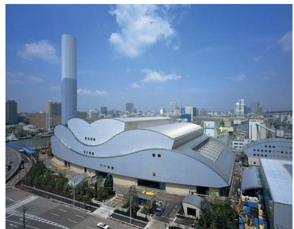
Tokyo – Minato EfW plant
