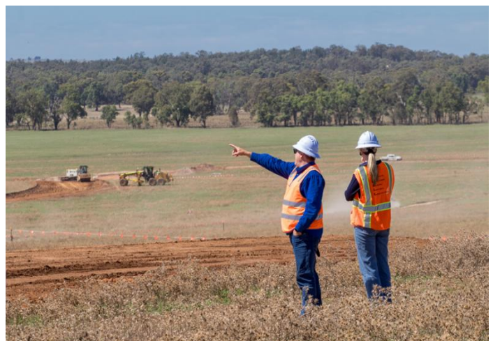
Pre-construction minor works at Merotherie
