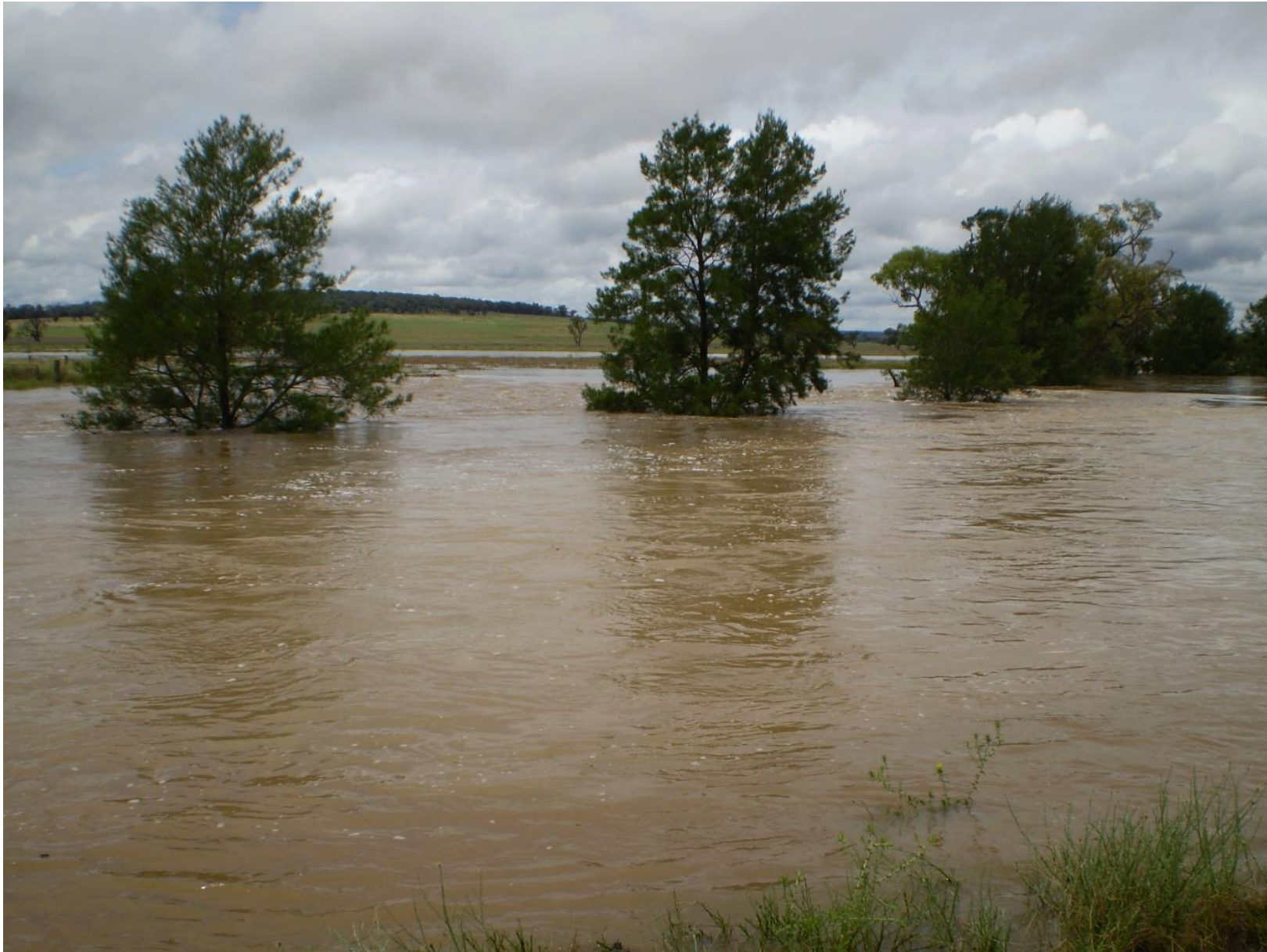
Talbragar River Bridge 5.12.2010
