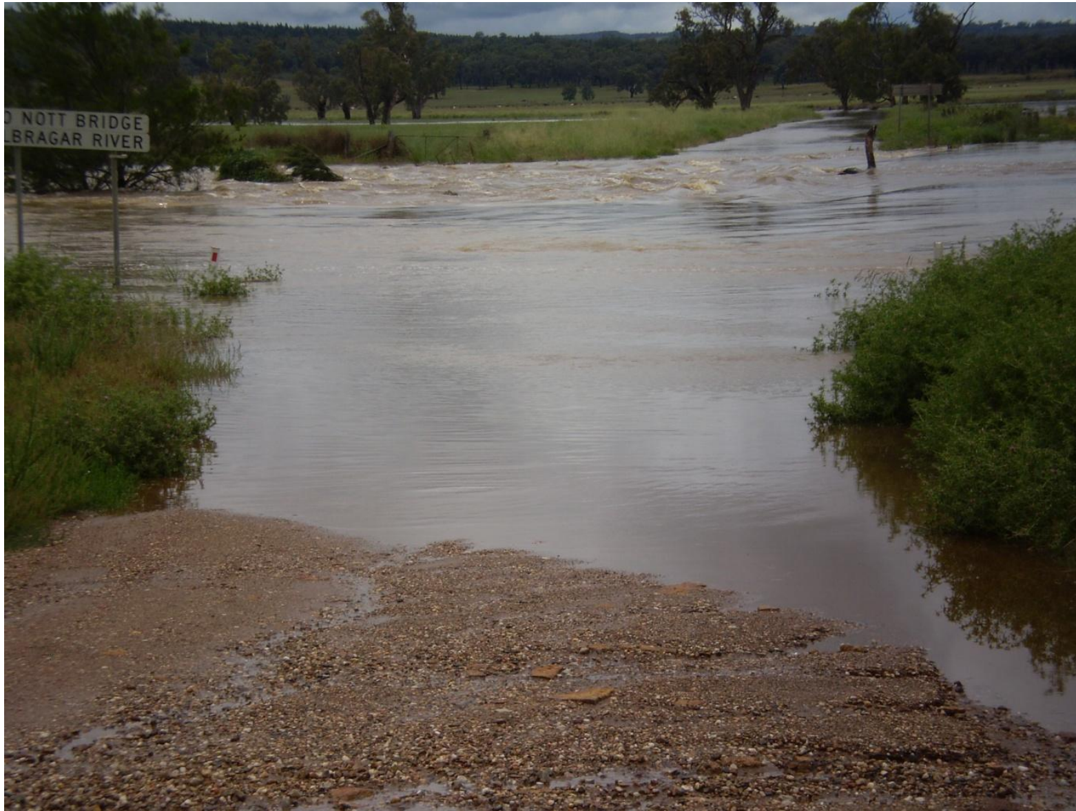
Talbragar River crossing Leo Nott Bridge 5.12.2010
