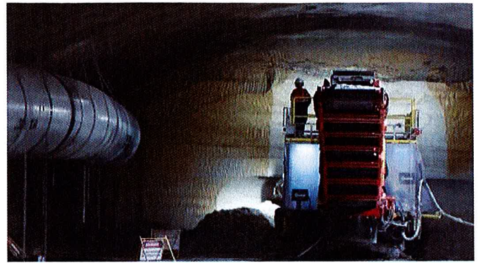
Roadheader excavation from the Cammeray site.
