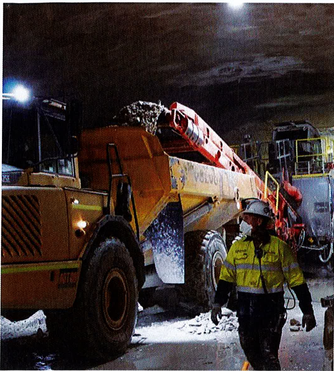
Roadheader tunnelling activities at Cammeray
