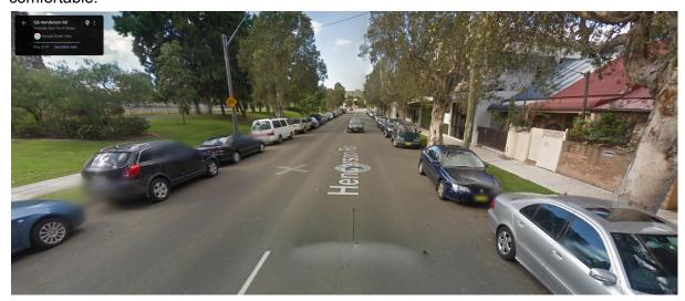
With the addition of the cycleway (shown here in Apr 2021) the driving area was narrowed to about 5 metres. The result is an environment where 50 km/h would feel quite uncomfortable, encouraging drivers to reduce their speeds closer to 30-40 km/h.
