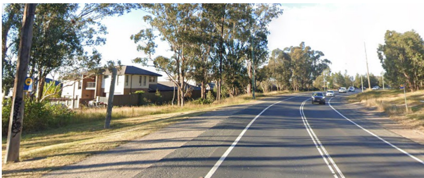
Figure 25 Example of typical rural-style road servicing a residential area in Cranebrook with no footpath, safe crossing point or bus shelters
