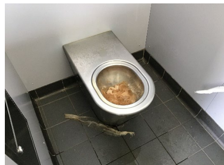
Figure 9: Branxton Truck Rest Area, Hunter Expressway
