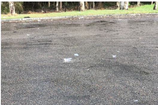
Figure 11: Wyong Service Centre N/B, Sydney-Newcastle Freeway
