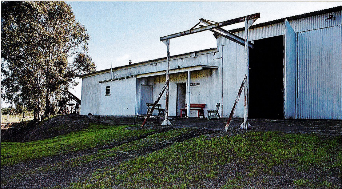
LOST: The shed on the Hatch family's property has stood the test of time but the bypass will see it demolished to make way for the roadway.
