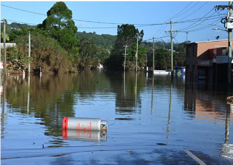
Figure 3 Images of flooding and damage around Lismore during and after the 2022 flood events
