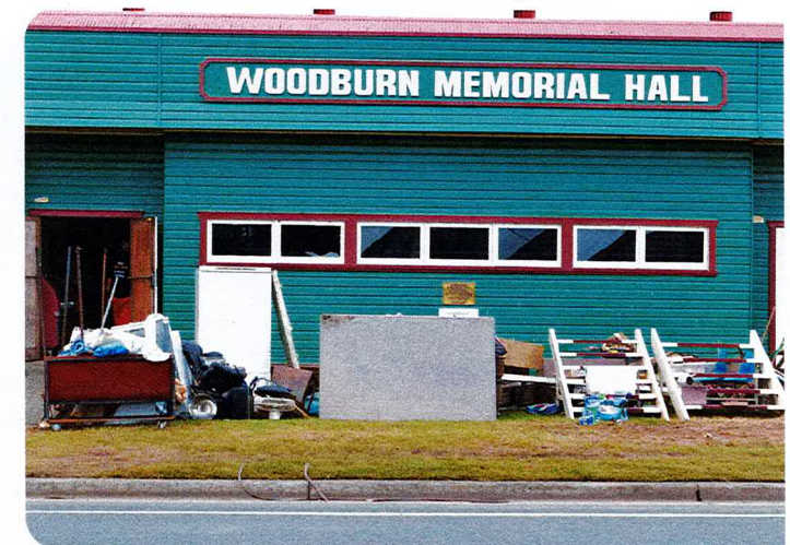
Flood damage at Woodburn Hall
