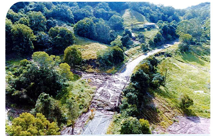
Naughtons Gap Road landslip
