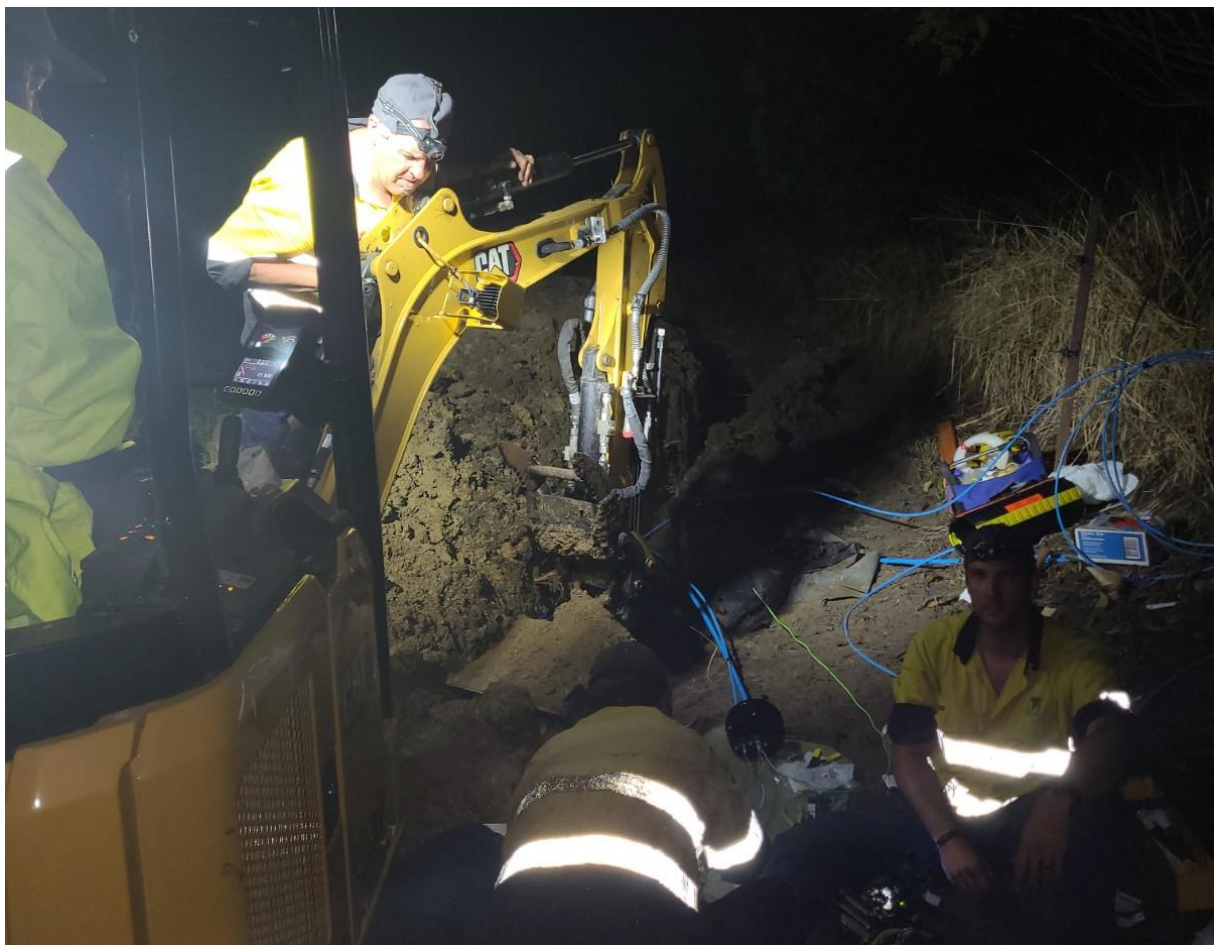
Restoration of fibre optic cables damaged in the 2022 floods.
