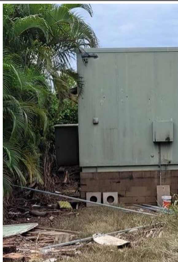
Figure 3: Exterior of Tumbulgum Exchange, showing mains power connection box located on the building wall on the RHS of the picture.
