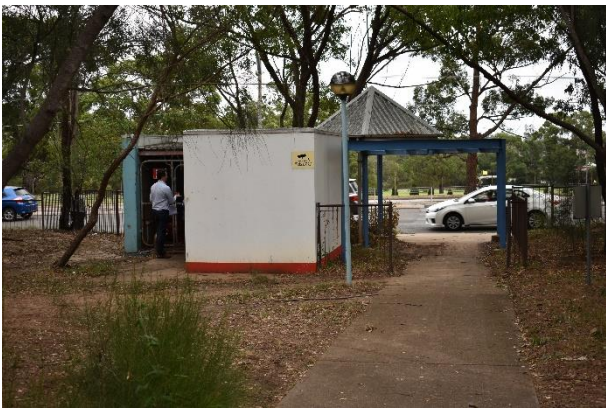
Picture 5 – Joseph Street bus stop from site
