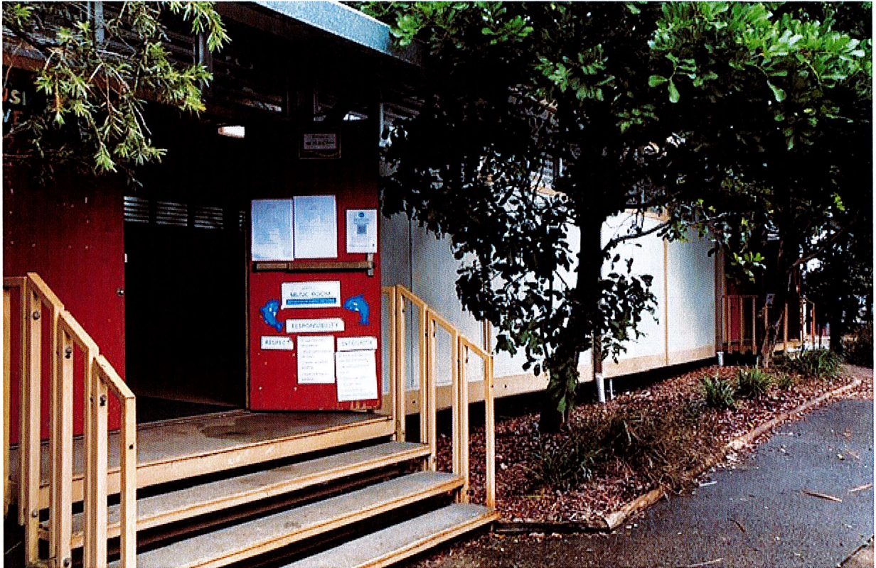
Canteen and music room located in a portable - exterior image
