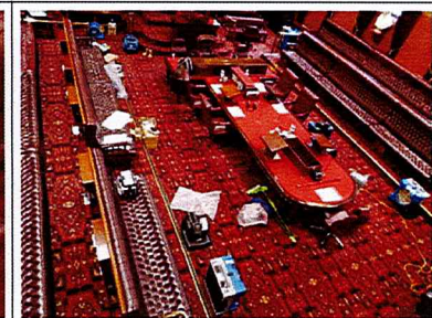
Photo 6: LC Chamber, equipment running during remediation works
