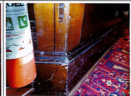
Photo 6: LC Chamber, walls skirtings prior to remediation works
