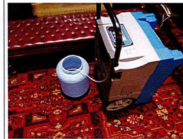
Photo 7: LC Chamber, Dehumidifier running during remediation works
