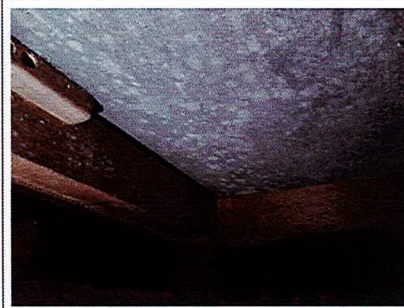
Photo 2: LC Chamber, seats underside prior to remediation works
