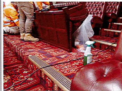
Photo 4: LC Chamber, during remediation works
