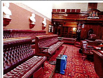
Photo 1: LC Chamber, overview followign remediation works
