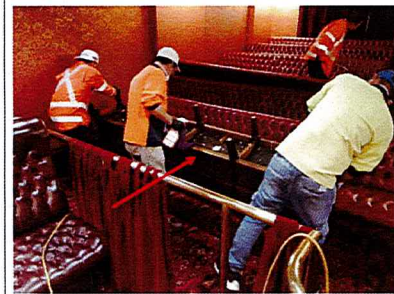
Photo 3: LC Chamber, during remediation works
