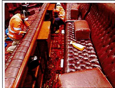
Photo 5: LC Chamber, during remediation works
