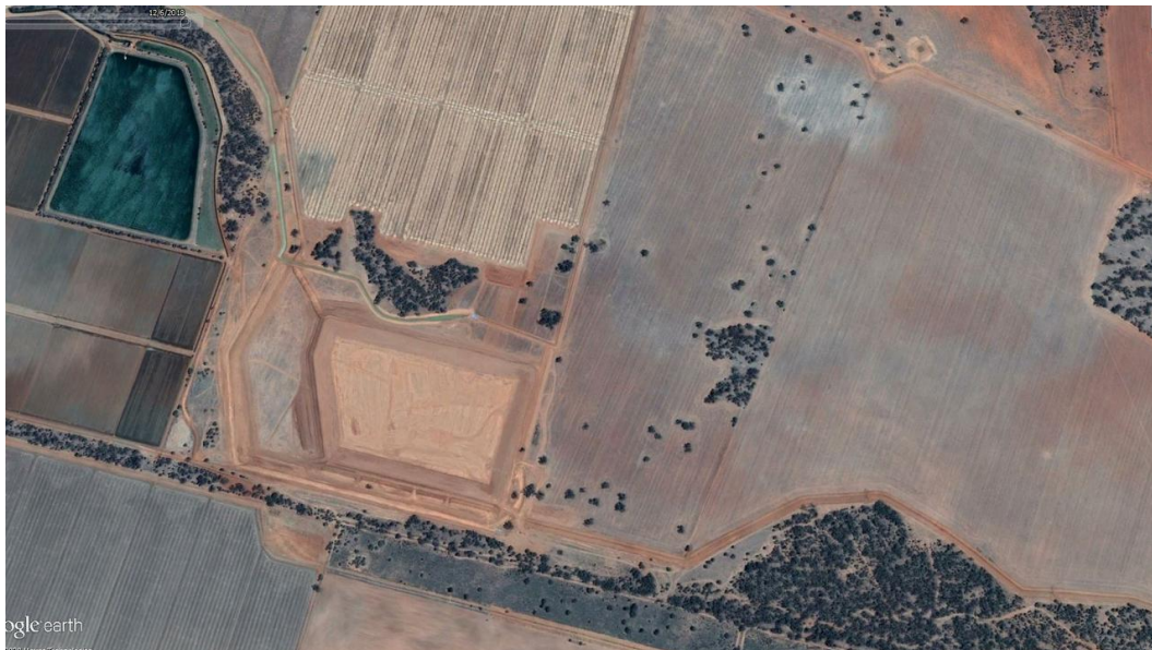
NSW state MP Helen Dalton's property after a new 785ML dam was constructed.
