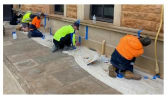
This conservation program included many trades required for a heritage building, including stone masonry, use of lime mortar not damaging cement mortar, carpentry, internal wall plastering, lathe and plaster ceiling repairs by adhesion, painting.
